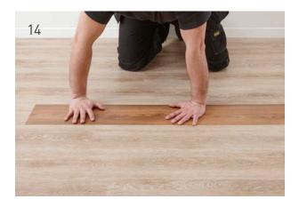
Push the replacement plank all the way down;
