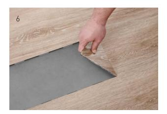
Pry the first plank section loose by inserting a putty knife in the cut running down the center of the plank. Gently unclick the first plank section from the adjoining planks;
