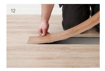
Insert the replacement plank at the short end by clicking it into the tabs of the plank already on the floor;
