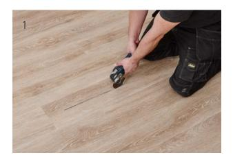
Adjust circular saw to the depth of the LVT board and cut the plank lengthwise along its center axis;
