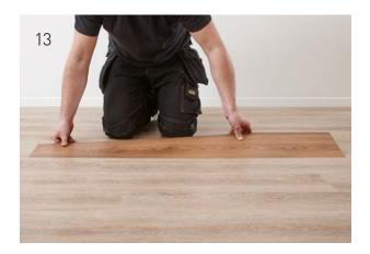
Fit the plank into the tabs at the other short end of the opening created by flexing it into place;
