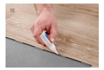
Remove the tabs on both long sides of the replacement plank; Leave the tabs on the short sides;
