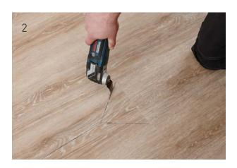
Carefully make radial cuts from the central cut to the 4 corners of the plank, making sure not to cut or otherwise damage the adjoining boards;
