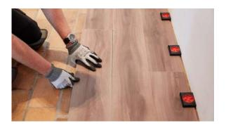
the correct fitting. Next, cut the panel to size. Doorjambs can also be sawn (undercut) to size if necessary, the LayRed 55 can them be neatly installed underneath.
